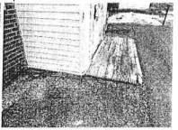
Failing brick sill at glass block wall
