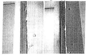
Numerous areas have visible water leaks which are shown by water stains on wood and ceiling
