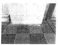
Head height does not meet current building code at base of stairs.
