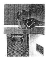
Handrail/guardrail at stairs does not meet current building code.
